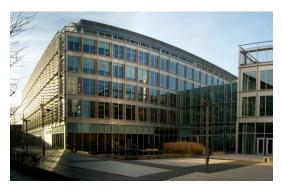
The Broadcast Centre is arranged over basement, ground and five upper floors. The fifth floor is set back from the building line and there is an additional sixth/roof level utilised to accommodate plant equipment. The building is of frame construction with metal-framed windows and provides high quality open plan office accommodation with a three-atrium design. In addition to this, the building incorporates areas of bespoke BBC operational equipment. The basement
