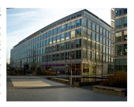
The Energy Centre is also of frame construction and effectively comprises two buildings contained within one envelope. The larger of the two sections houses the plant requirements for Broadcasting Centre and Media Centre. The smaller section offers potential office accommodation which is currently unoccupied and in a shell condition.
