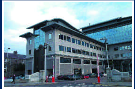
Talisman House Aberdeen
