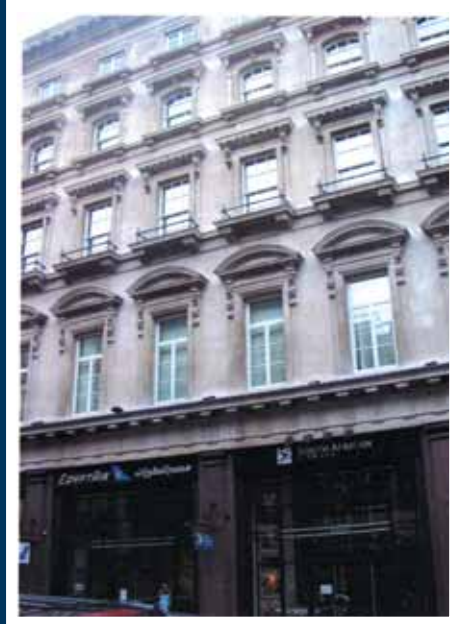
St George's House, London Podium & St George's House
