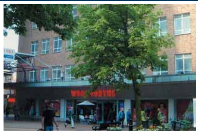
49 The Precinct and 2-12 (Even) Market Way, Coventry Market Way
