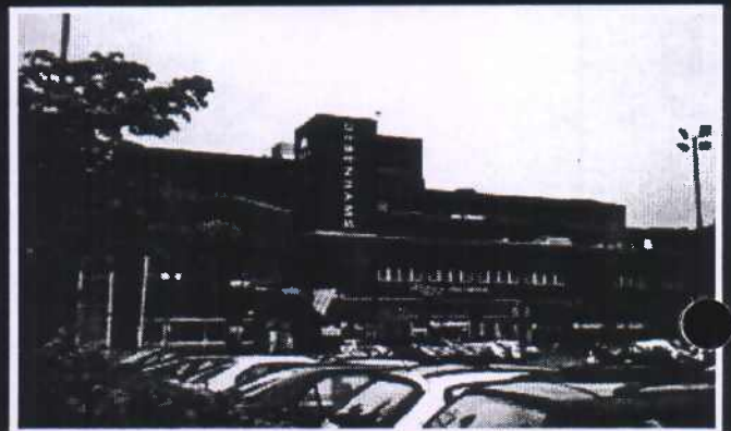
Fishergate Centre Preston
